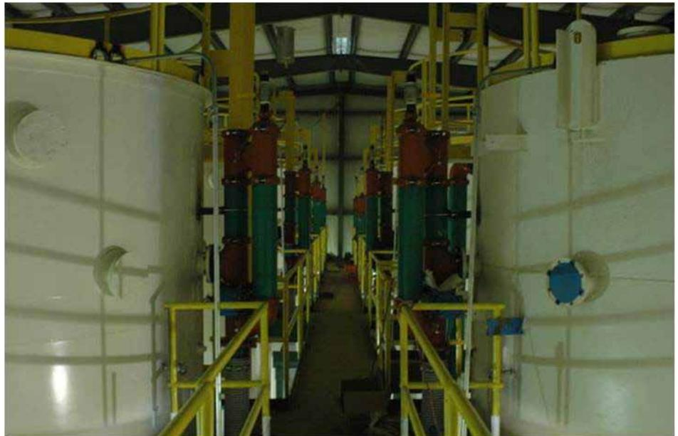
When complete and in full operation in early 2011, the Hampton Feed Lot anaerobic digester will create methane gas in tanks like the ones shown above and will burn it to produce up to 14,400 kilowatt hours of electricity per day. Located in Chariton County, Hampton Feed Lot regularly houses approximately 2500 head of cattle.
